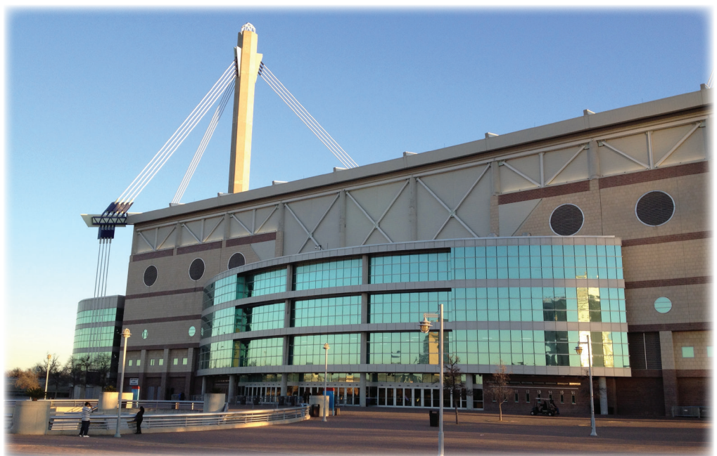
Alamodome, San Antonio, Texas, USA (photo courtesy of ANN)
